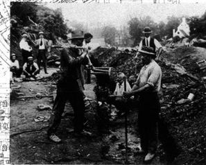
33rd Street Construction, 1914
